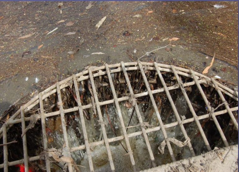
Clogging of wetland outlet structure
